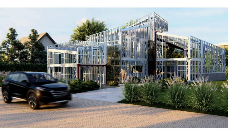
Thanks to its excellent strength-to-weight ratio, the amount of material required to build the same surface is significantly reduced.
